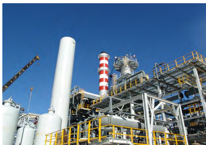
A hydrogen plant refinery under construction (Photo: Shutterstock)
