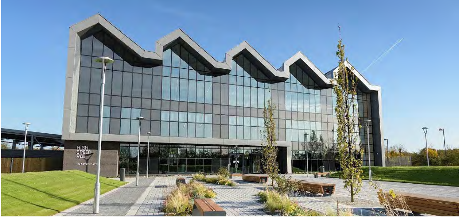
National College for Advanced Transport & Infrastructure, Doncaster.
